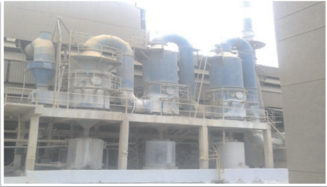
HCL Fumes Scrubbing System for Fertilizers Complex
