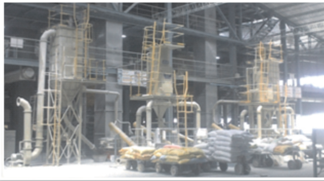
Dust Collection System for Raw Material handling complex of a Detergent Factory
