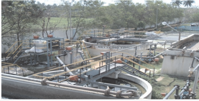
Effluent Treatment Plant for FMCG customer
