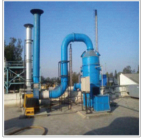
FUME SCRUBBING SYSTEM
