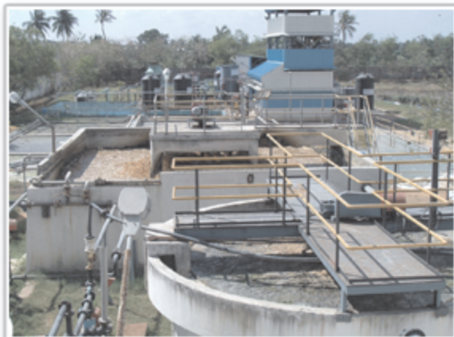
EFFLUENT TREATMENT PLANT
