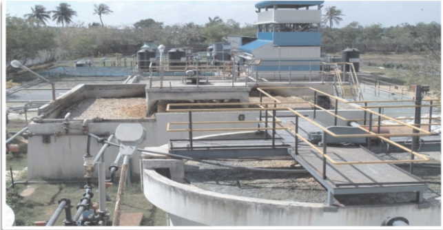
Effluent Treatment Plant for FMCG customer
